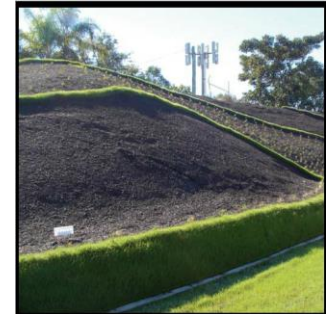
Slope Protection and Erosion Control Blanket
