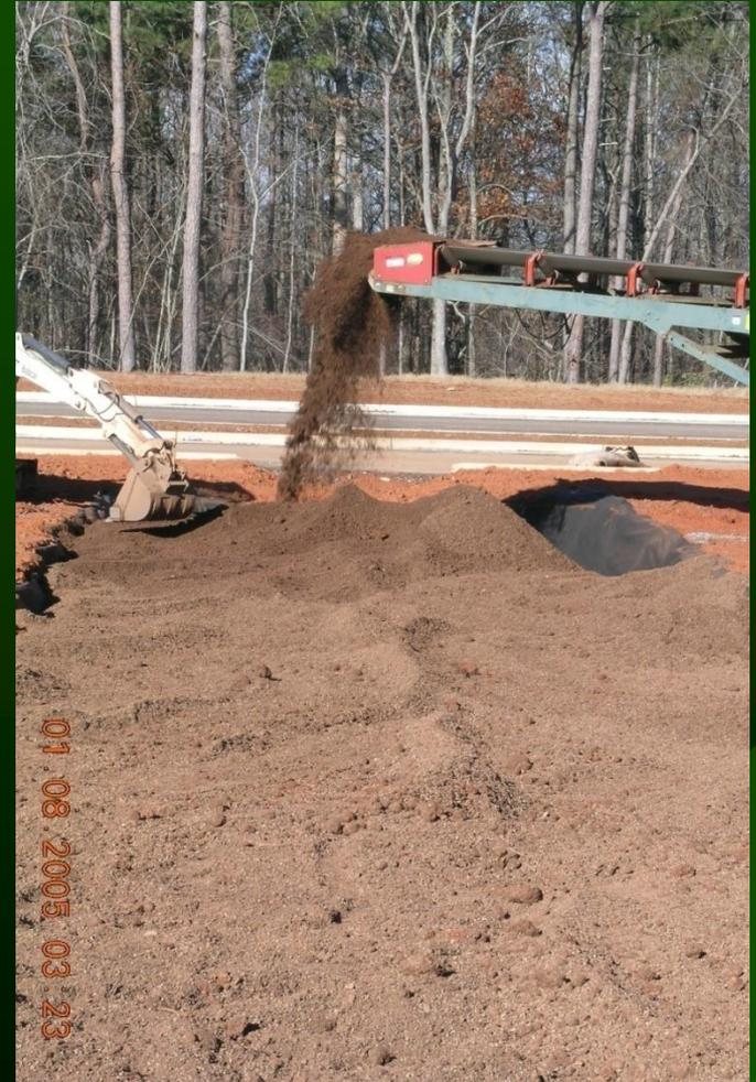
Conveyor or Blow Soil Into Place to Alleviate Over-Compaction
