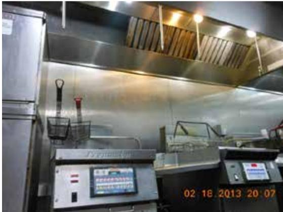
2. Hood # 1 and Baffle Grease Filters (# 0338)
