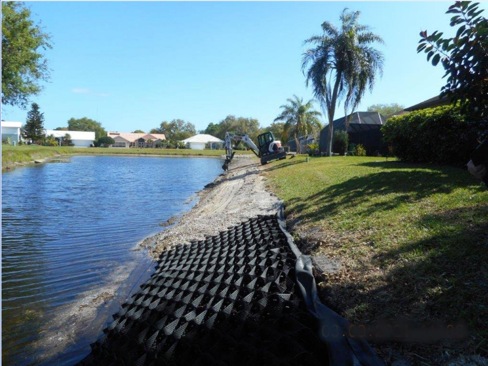
***Geoweb reinforced banks (\$100–\$150 per linear foot)***
